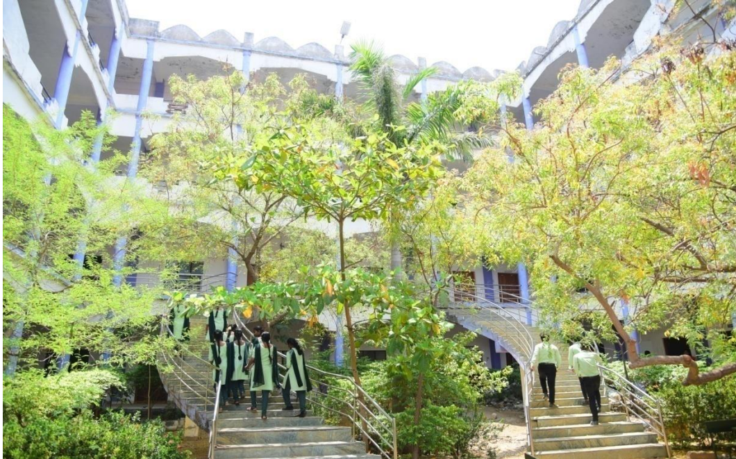
Civil Block in PSNEC
