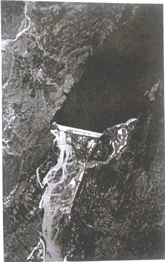
Satellite image of Tarbela Dam on the Indus River in Pakistan (Courtesy, Johnson Space Center, NASA)
